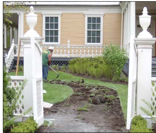
Path at southwest corner of formal garden, under construction, May 2005.
