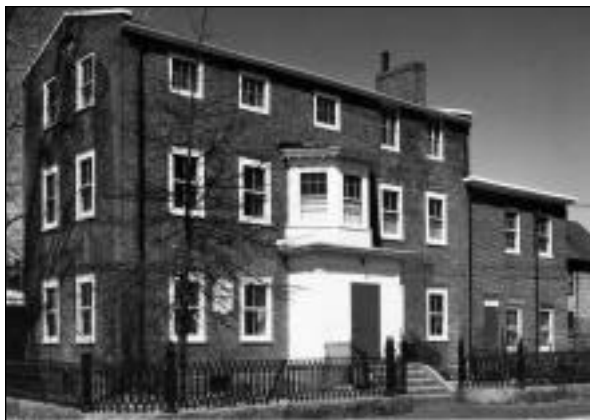
Cambridge Neighborhood House, 79 Moore St., demolished 1973
